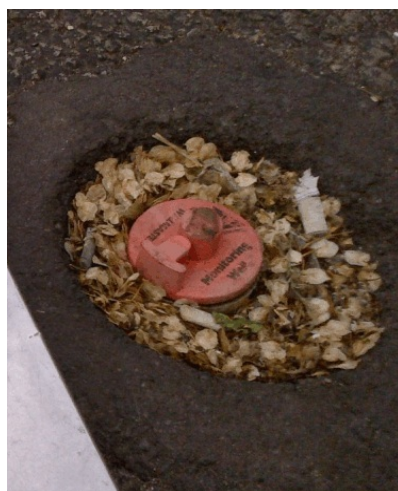
The casing for this well has been lost - the cap is now vulnerable to physical damage, and surface water or spills will pool around it, waiting for a weakness.
