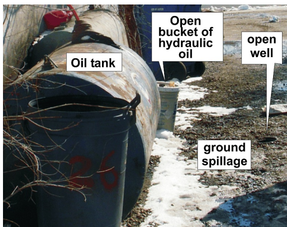
A damaged and open well plus multiple nearby contaminants means that groundwater at this property will soon be affected. Ironically the well was originally installed to demonstrate that the property is clean.
