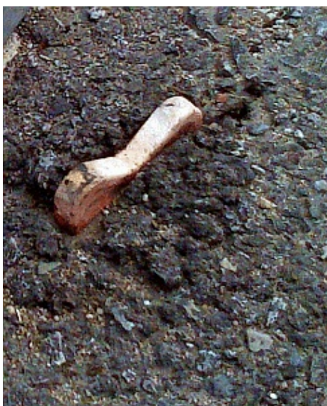
The casing for this well has been lost - the cap is now vulnerable to physical damage, and surface water or spills will pool around it, waiting for a weakness.
